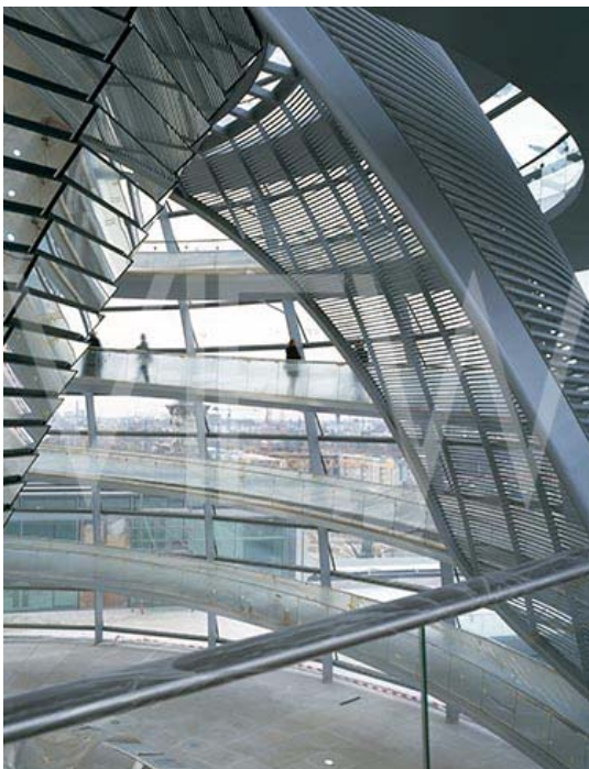
Fig. 6. The dome of a daylight on the German Parliament ( www. German Parliament )
